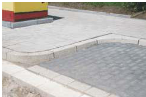
Granoment Pflaster 10/20/8 in Quarz 0-5 mm und Basalt-anthrazit 0-5 mm
